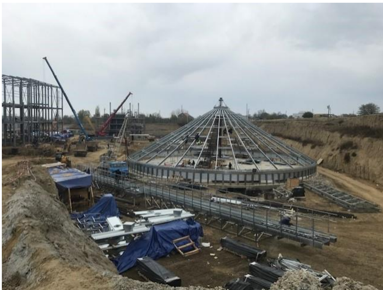
Figure 64: Construction of the modern sunflower oil factory within the GIFP Business Park (2020).
