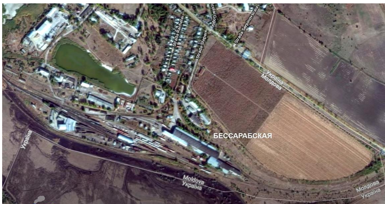
Figure 29: Junction railway station Basarabeasca
