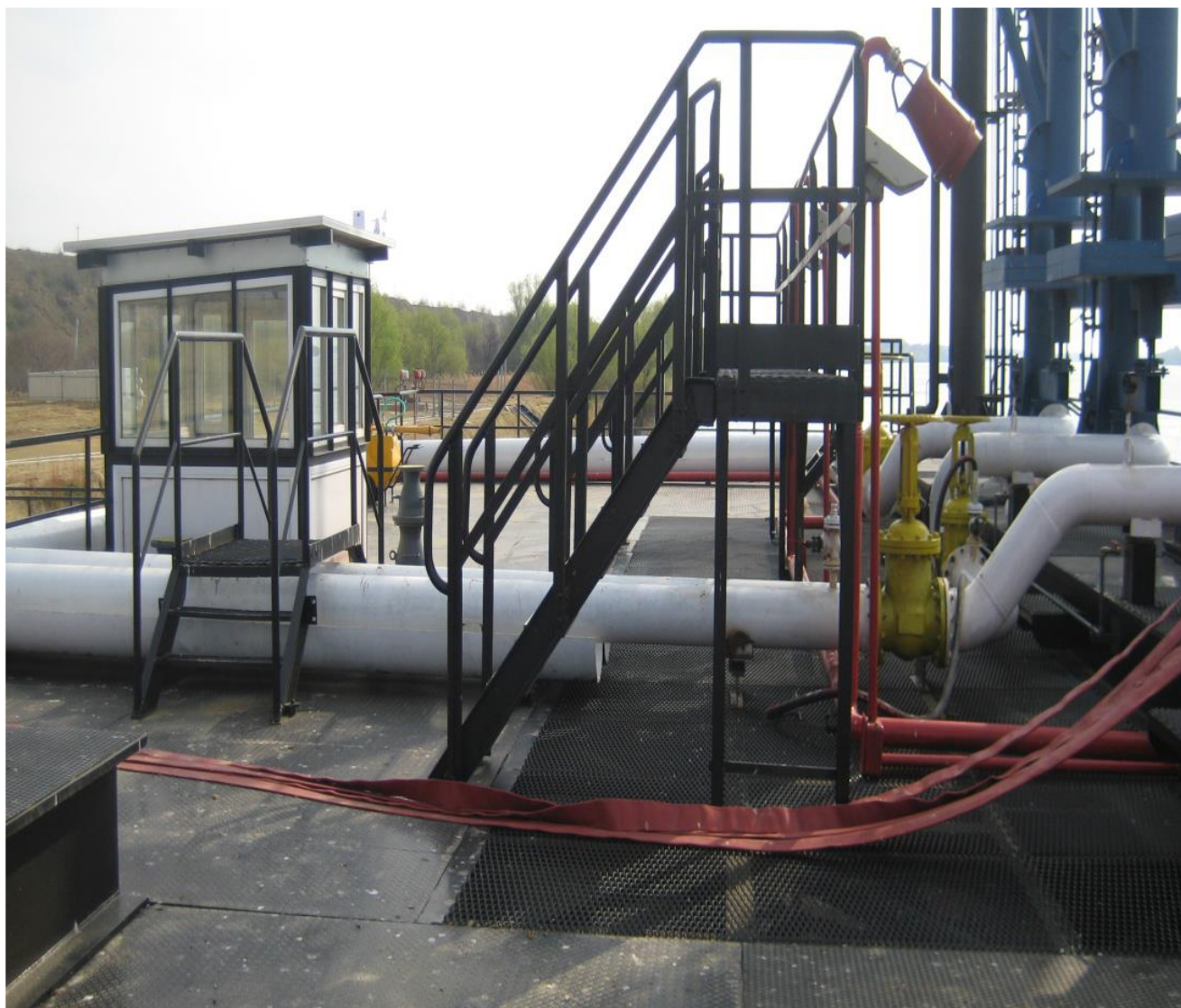
Figure 61: Oil transfer equipment
