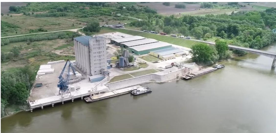
Figure 6.8. Port of Bogojevo existing grain terminal with two berths
