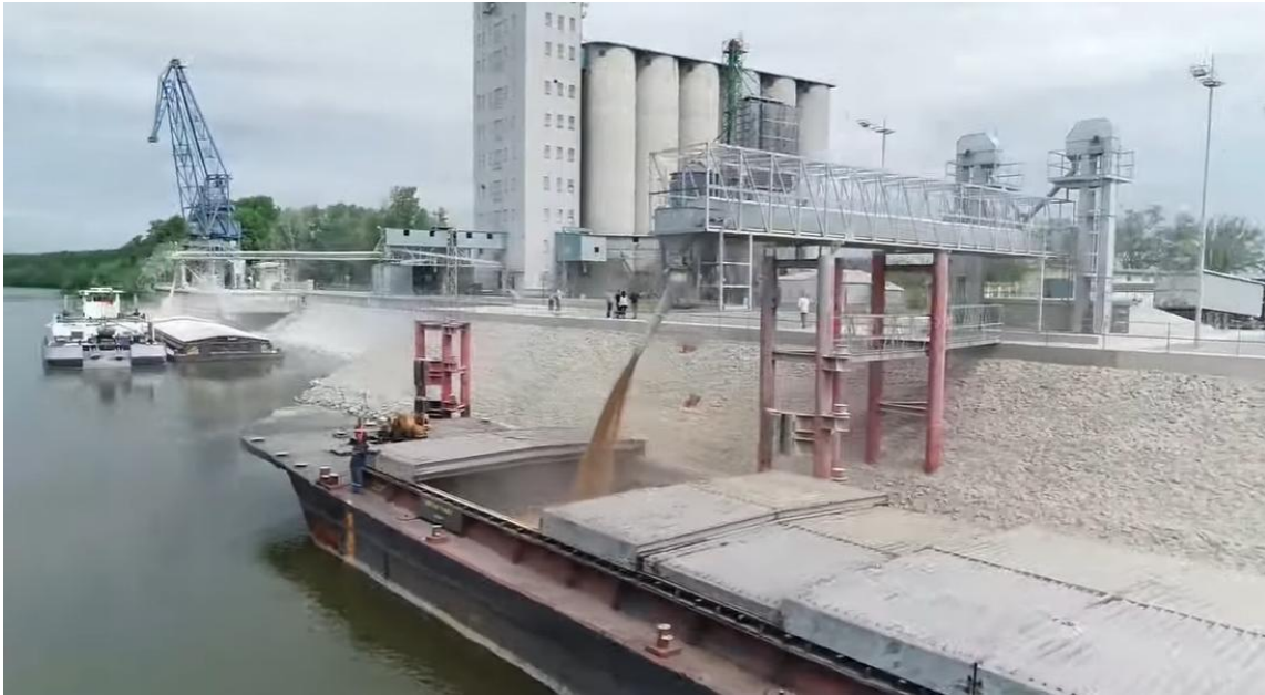
Figure 6.9. Grain loading facility at the sloped quay
