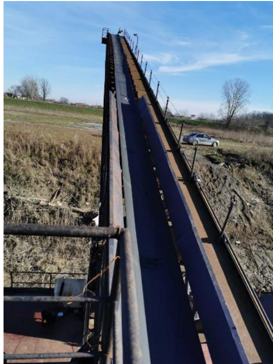
Figure 6.3. Belt conveyor for the transport of gravel from the bucket elevator to shore
