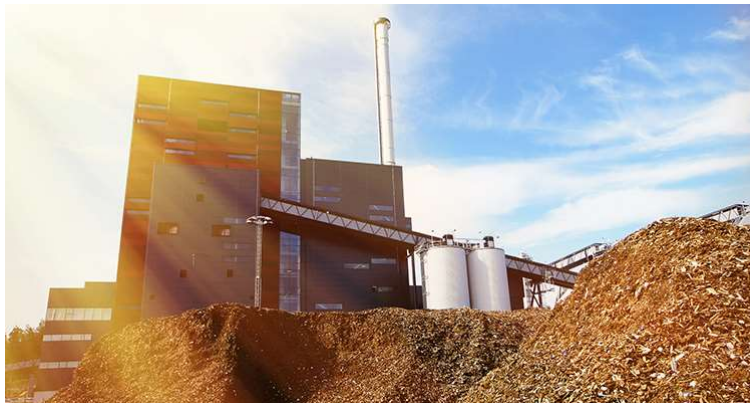
Figure 5: Bioelectric plant with woodchip storage
