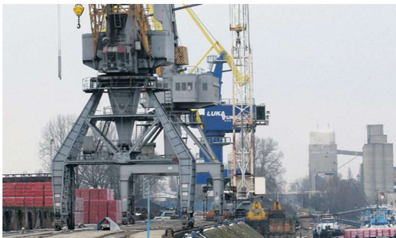
Figure 4: Cranes in the port of Vukovar
