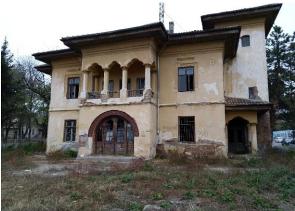
Figure 11: Ex- water police station 2022
