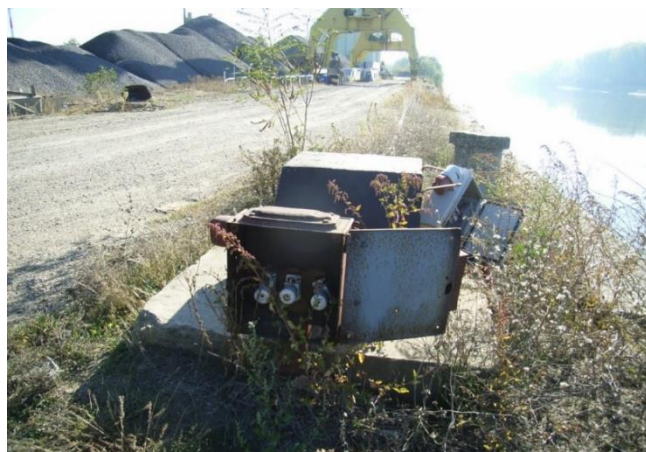
Figure 8: Non-functional electric switch box
