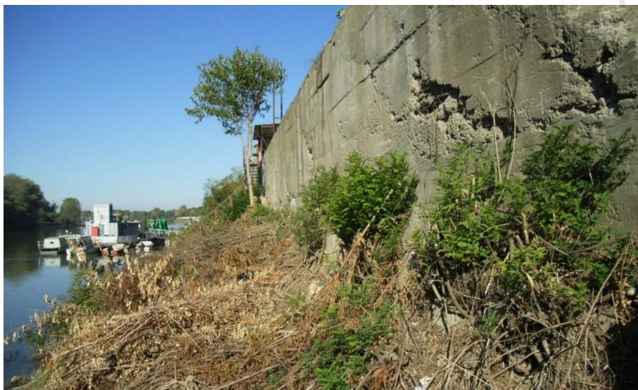
Figure 4: Vegetation at the base of the vertical quay
