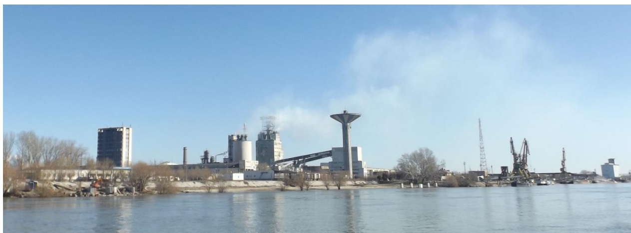
Figure 14: View of Turnu Măgurele Port from the Danube
