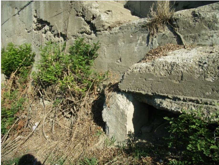
Figure 5: The foundation of the vertical pier
