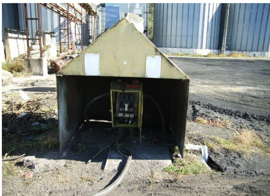
Figure 24: Degraded electric switch box
