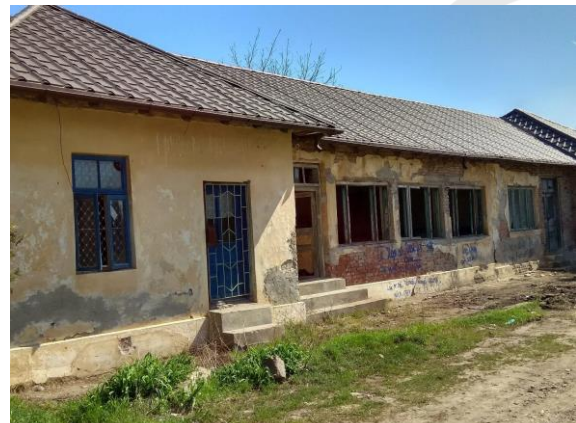
Figure 12: Ex- port railway station 2022
