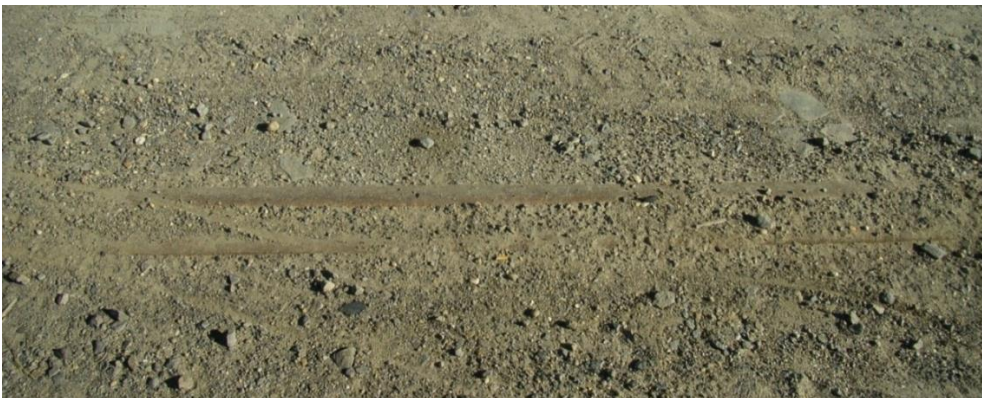
Figure 7: Rails covered by deposits
