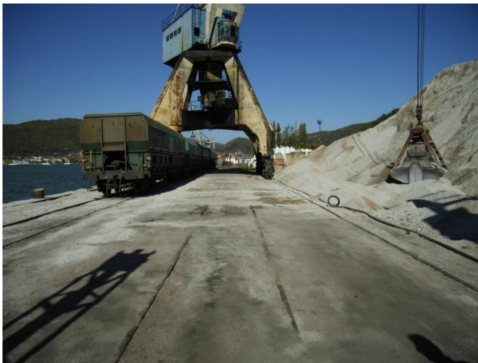
Figure 23: Railway in the northern zone
