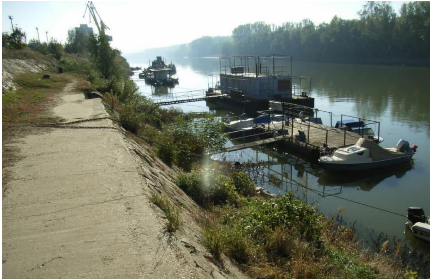
Figure 3: Vegetation on the revetment
