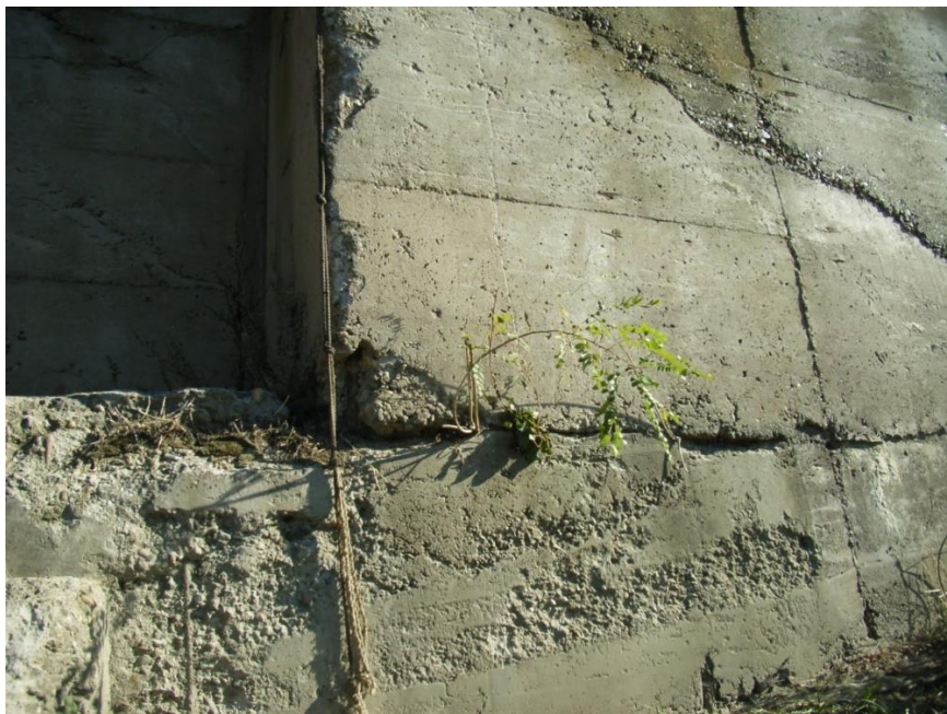
Figure 6: Cracks and exfoliations on the face of the vertical pier
