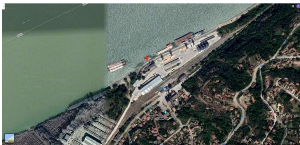
Figure 22 Port terminal Somovit
