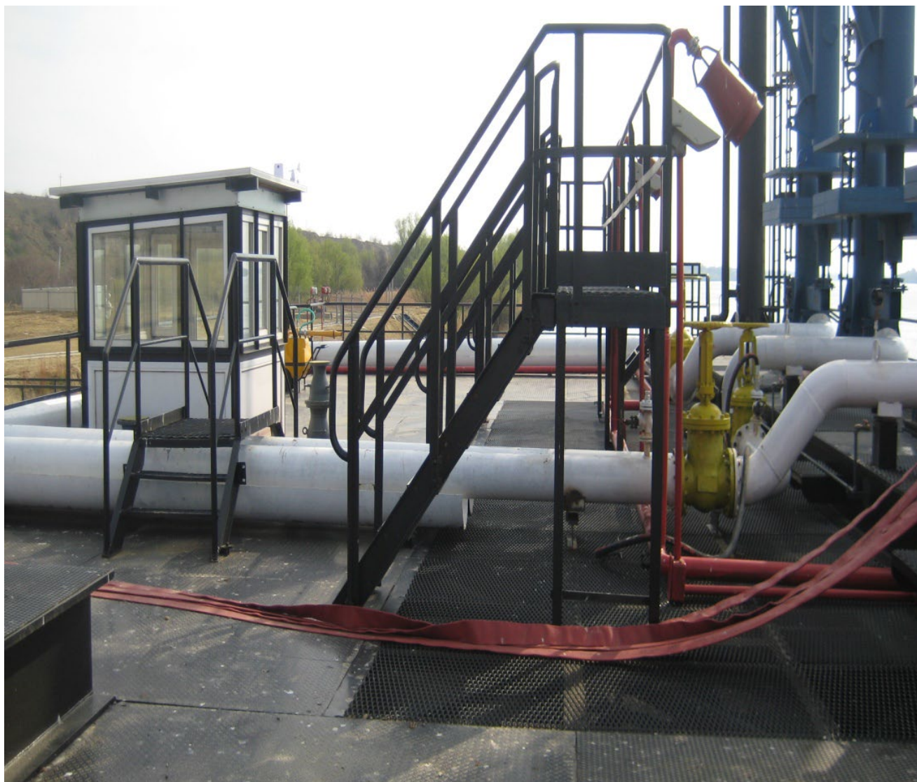
Figure 50: Oil transfer equipment
