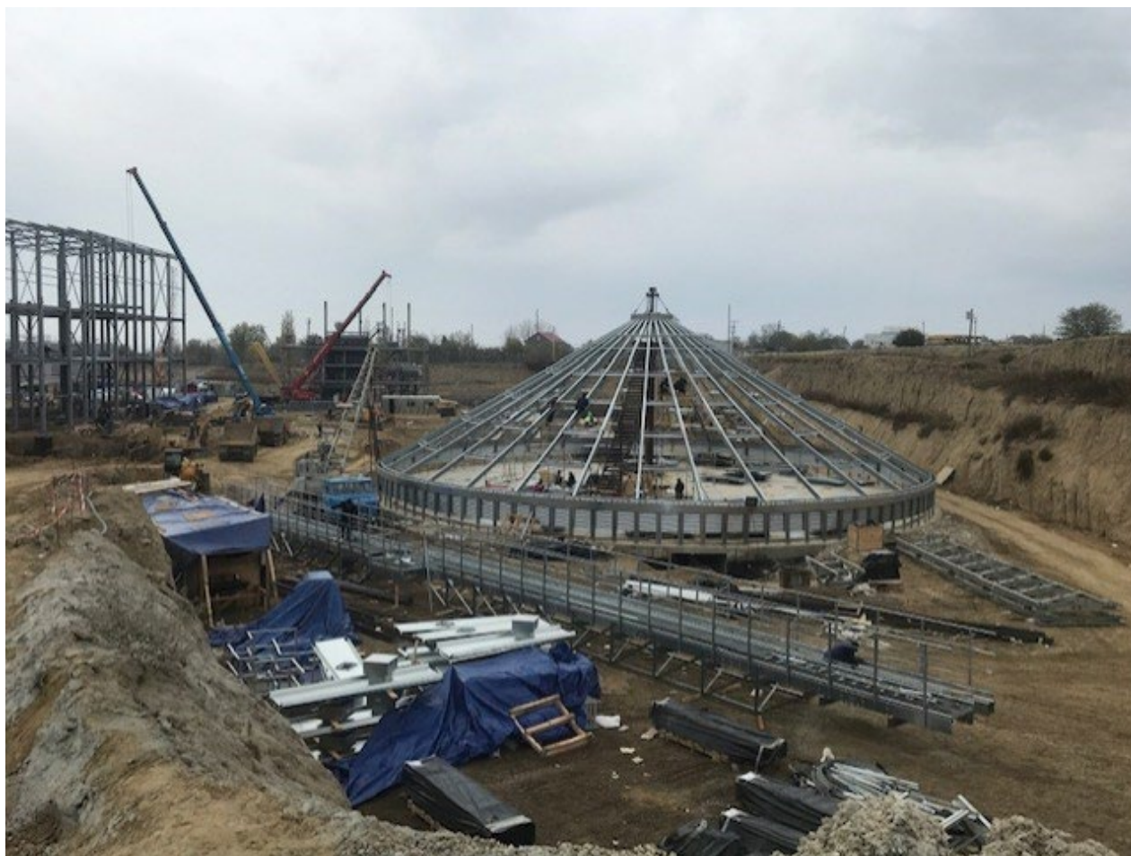
Figure 53: Construction of the modern sunflower oil factory within the GIFP Business Park (November 2020).
