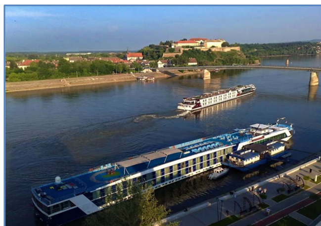
Figure 10. IPT in Novi Sad - DP World Novi Sad docking facility
