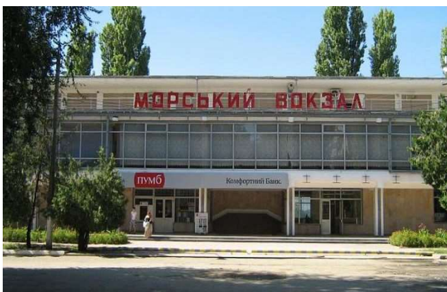
Figure 1. Passenger terminal of Reni seaport
