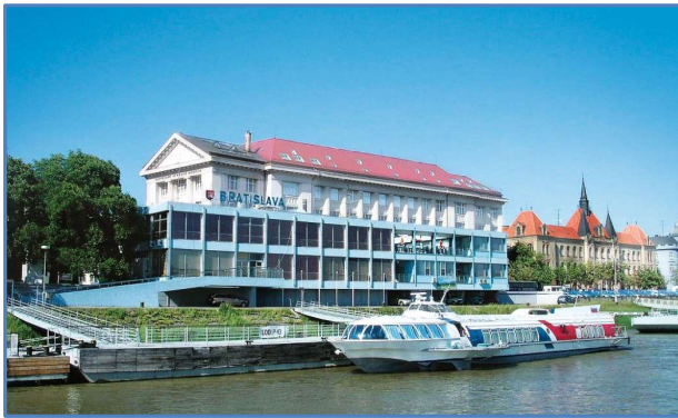
Figure 4: Passenger terminal Bratislava
