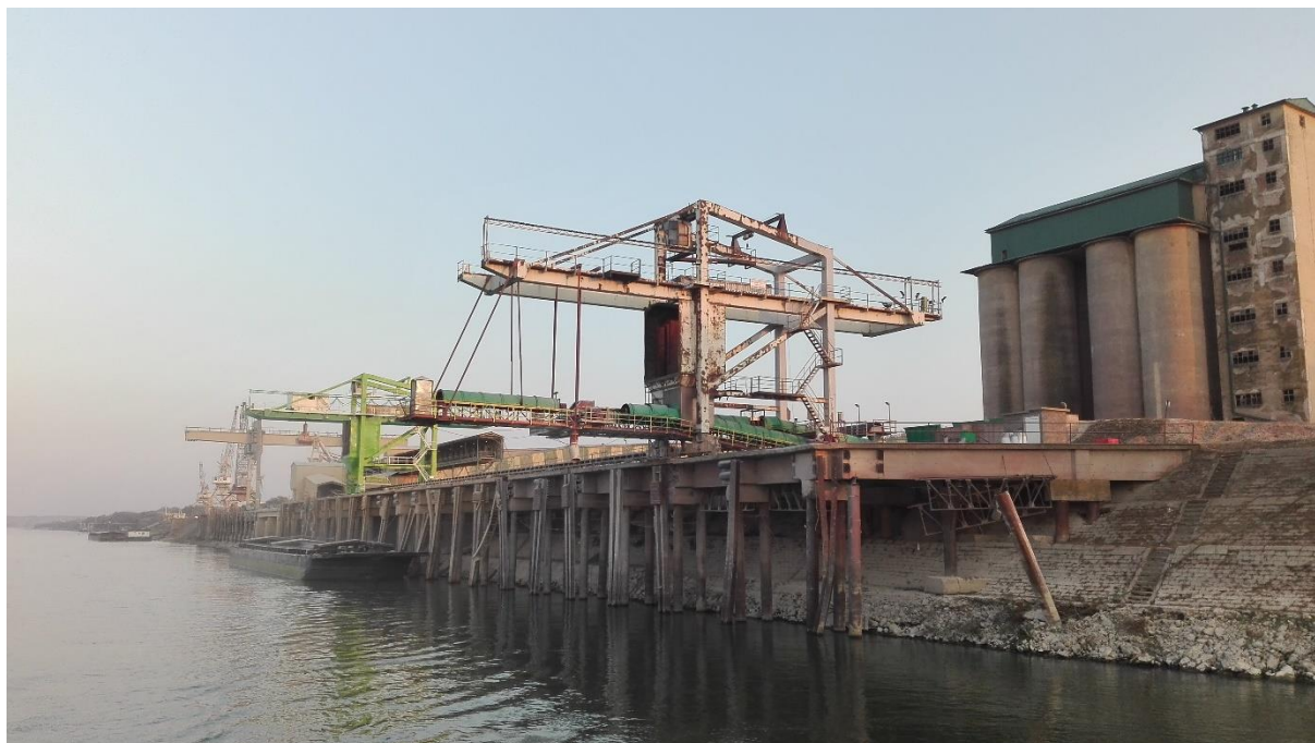
Figure 25: Port of Prahovo
