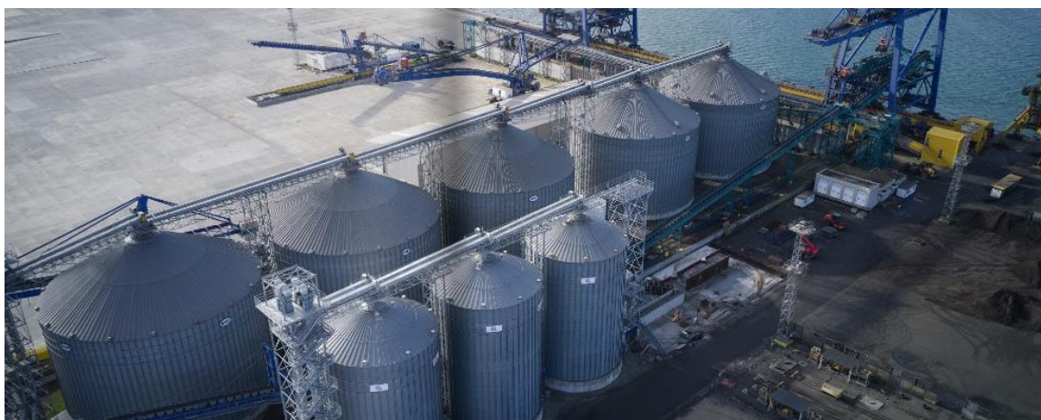
Figure 67: Silo complex in port terminal Burgas East 2
