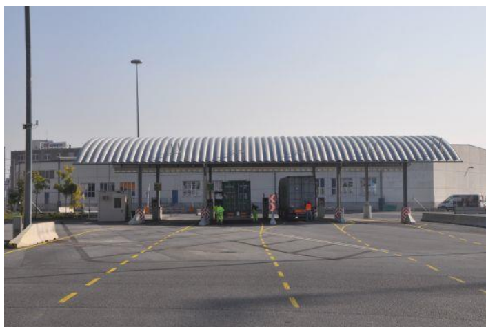
Figure 59: Foto-IN-Gate-Entry at the container terminal of the Port of Vienna 45
