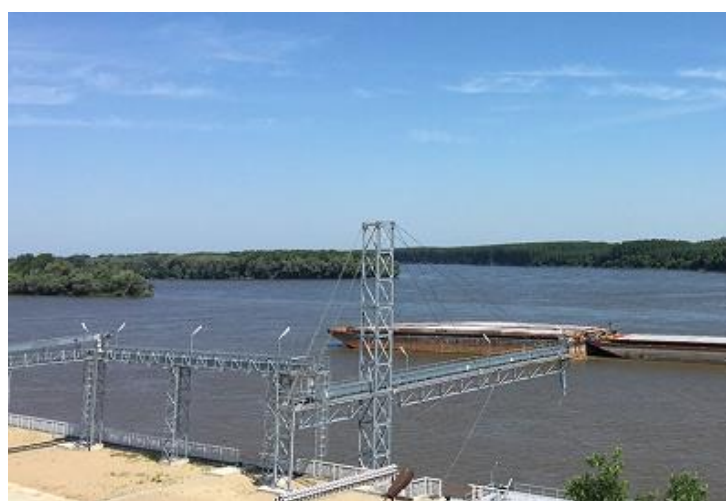
Figure 92: Cantilever metal construction for grain loading
