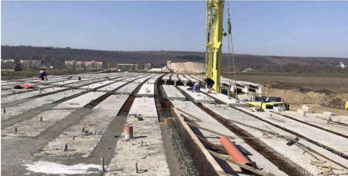
Figure 31: Construction of the Comrat bypass road
