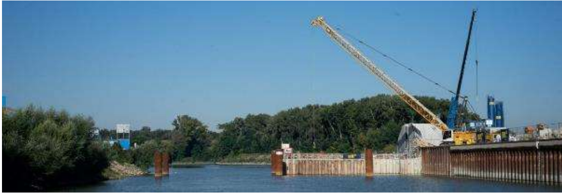
Figure 4: Construction of Port Gate (Port of Vienna) 6
